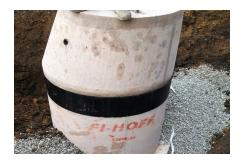
For this sewer line extension, the manholes along the force main required protection from microbial induced corrosion. Liners or coatings would normally be used to perform this function. As these are expensive and time consuming to install, the engineers decided to specify the inclusion of Xypex Bio-San C500 admixture in the pre-cast concrete.
